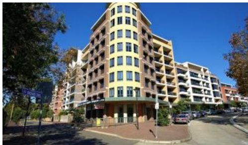
Unit 118, 1 Brown St, Ashfield
