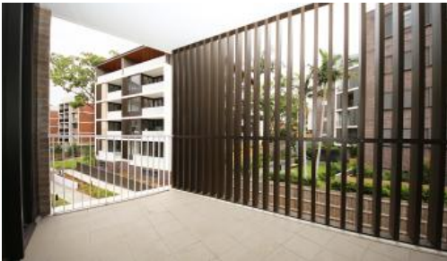
A302, 22 Birdwood Avenue, Lane Cove
